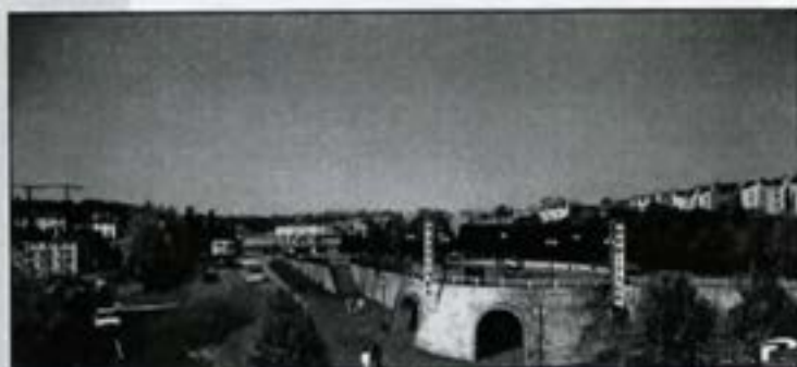
Station Approach – A design for the future
