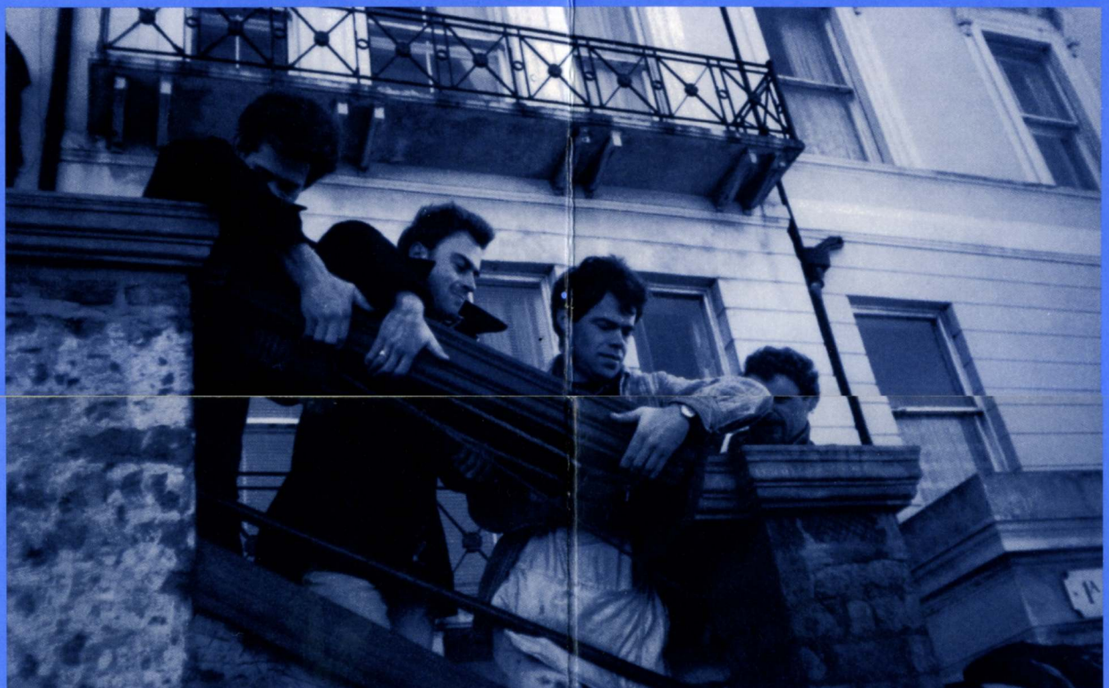
Wellington Square. Replacing broken balustrade.
