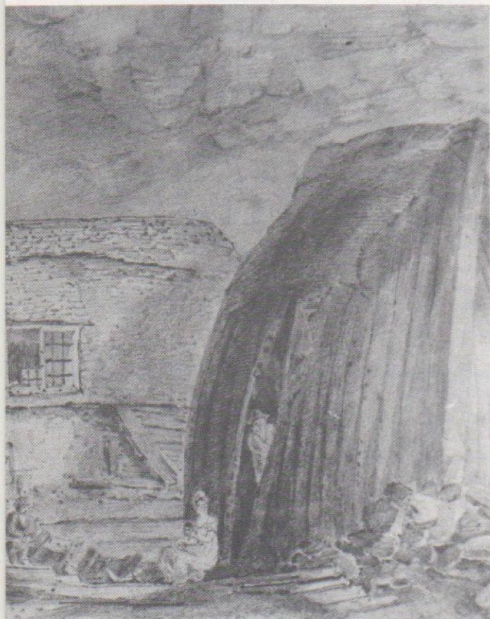
A possible originator of the net shops – an old boat has been cut in half, and up-ended as a store for nets and gear. As you can see, families sometimes also lived in these shelters. This drawing was made about 1820.
