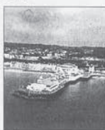
Sea view, damage done by salt water, and the cost of maintenance, are significant to the pier's owners. But the main point of the competition is to find new uses. These
