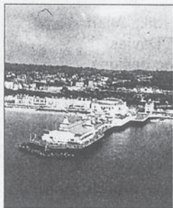
Sea view, damage done by salt water, and the cost of maintenance, are significant to the pier's owners.
