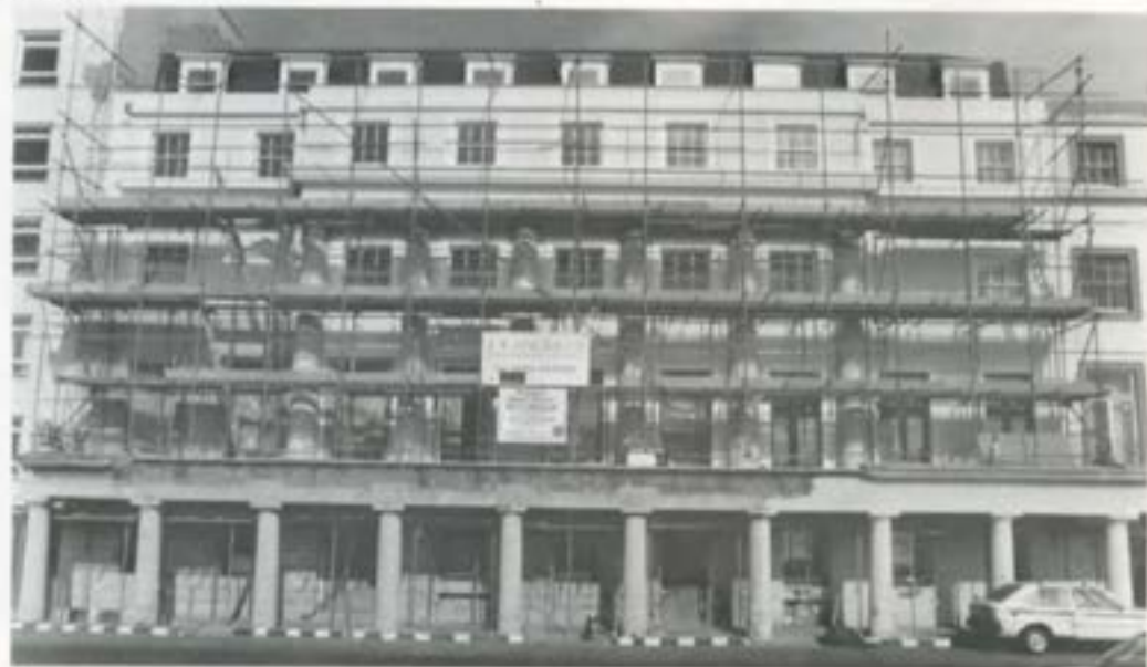
Conway Court, so near to demolition in 1986, is now nearing the end of an 18 month refurbishment programme.
