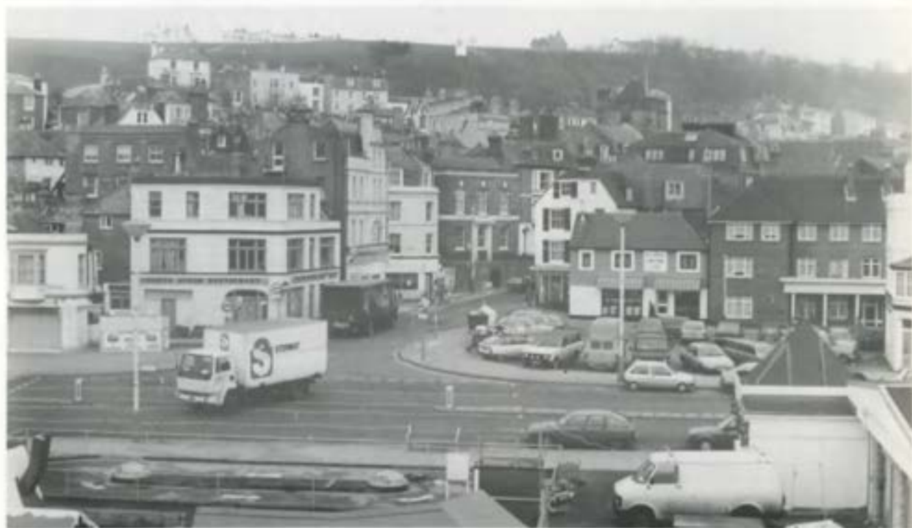
"Opportunities for Action": Environmental improvements, as here at the entrance to High Street, would make the main approaches to the Old Town more inviting.
